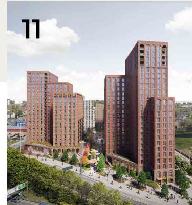
___ LEEDS URBAN VILLAGE, LEEDS
